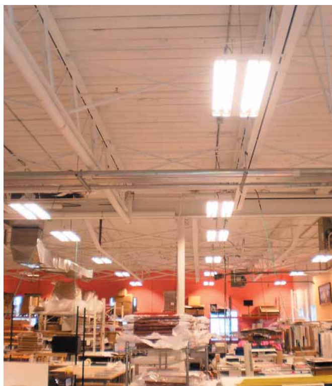
Lights mounted high in the ceiling of warehouses don't always work well for production operations. Lower fluorescent lighting can be used more effectively and is often many times more efficient for production lines and cells.
