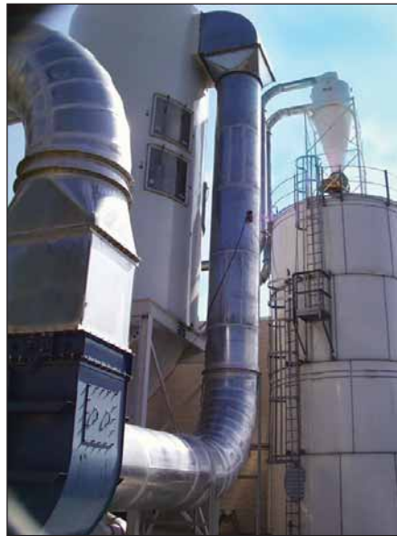
Larger framing manufacturers, such as the Framera plant on Long Island, use systems that collect dust and feed it to furnaces to heat the facility in colder weather.
