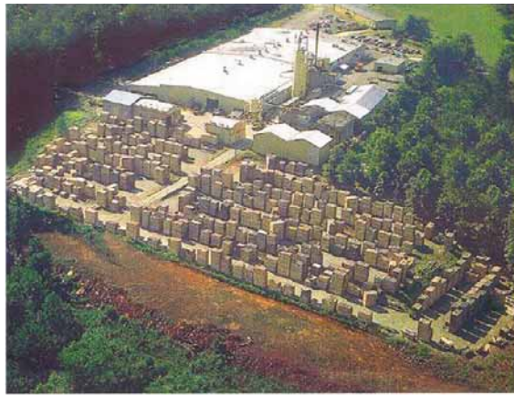
T.I. Industries' main finishing facility and lumber concentration area reflects the company's investment in its own forest to provide raw materials for moulding.
