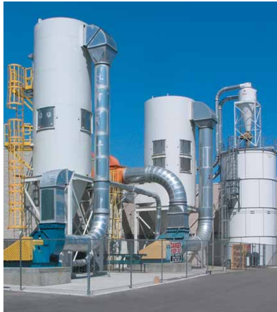
Framerica’s environmental efforts include a state-of-the-art dust collection system that recycles waste to heat the building.
